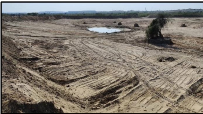
Nadi before completion
