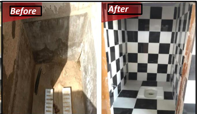
Upgradation of sanitation facility at schools
